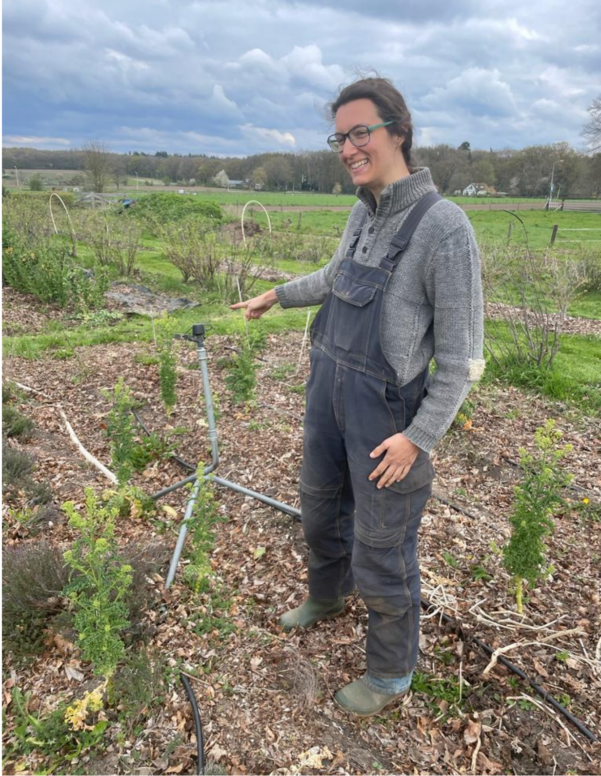
Figure: A sprinkler irrigation equipment
